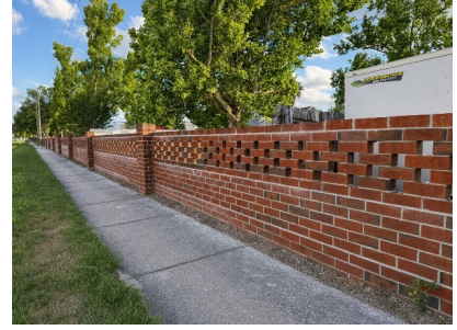
Completed: reconstructed, strengthened, and fully tuck-pointed perimeter wall.
