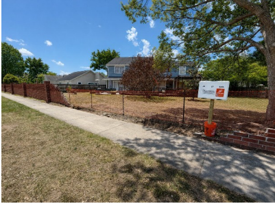
Demolition: failed wall sections removed and work area secured.
