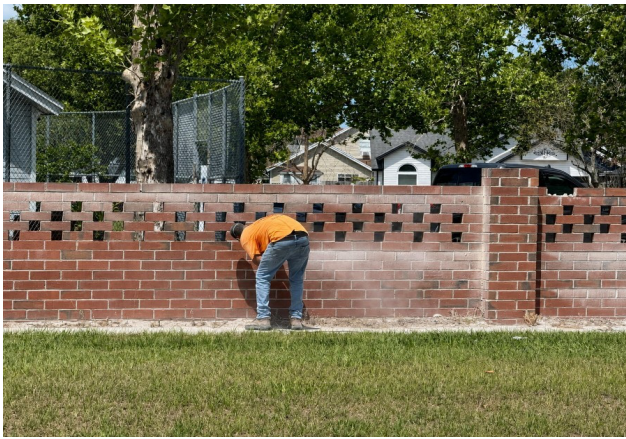
Tuck-pointing renewed deteriorated mortar joints across the existing wall.
