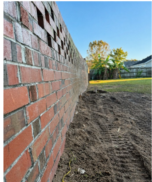
After vegetation and root-hazard removal, the wall corridor was cleared for inspection and maintenance.
