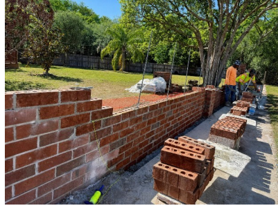
Reconstruction: new masonry, reinforcement, and alignment work in progress.
