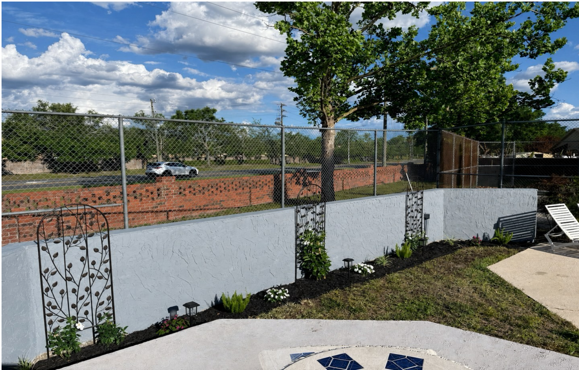
Restored gray pool wall with rebuilt planting beds, black metal trellises, new plantings, and landscape lights.
